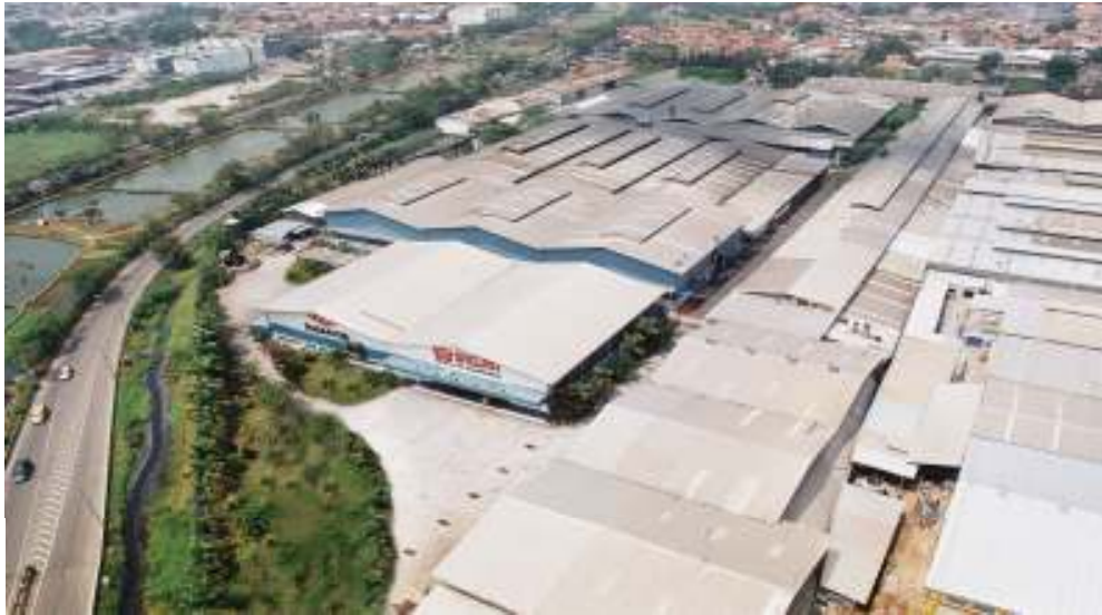
Kapuk Plant (Radiator Facilities)
